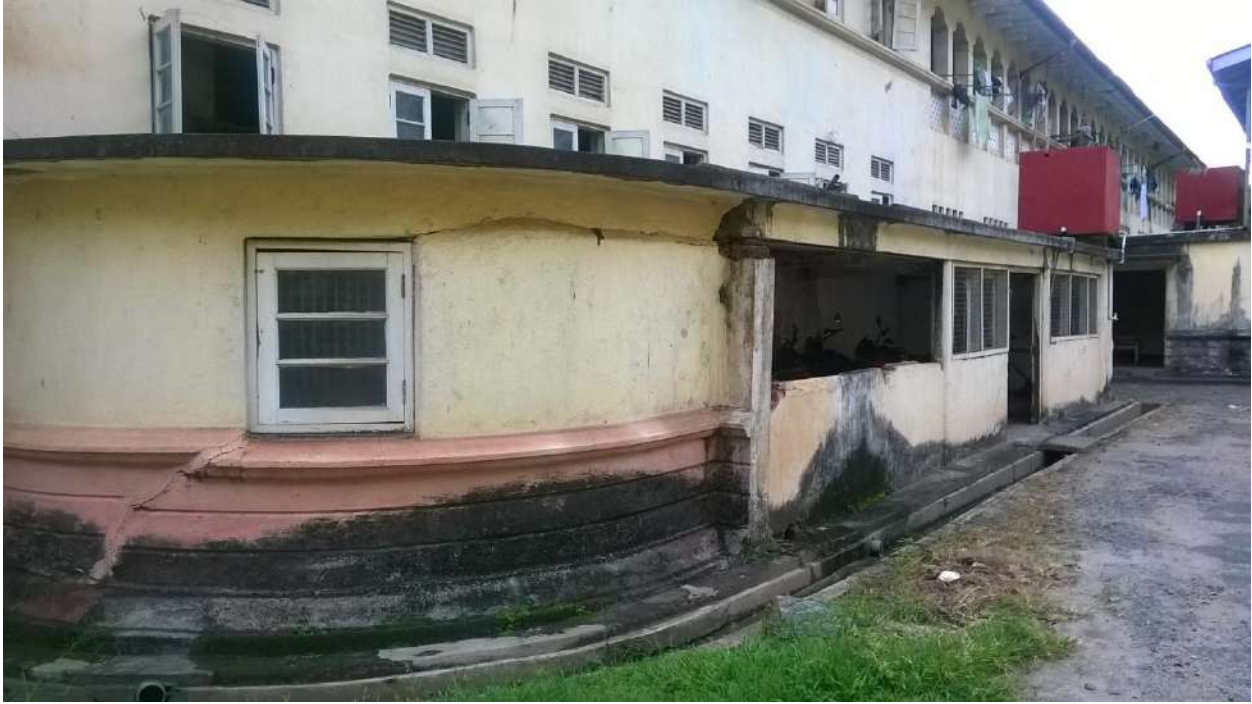
Existing cycle shed
