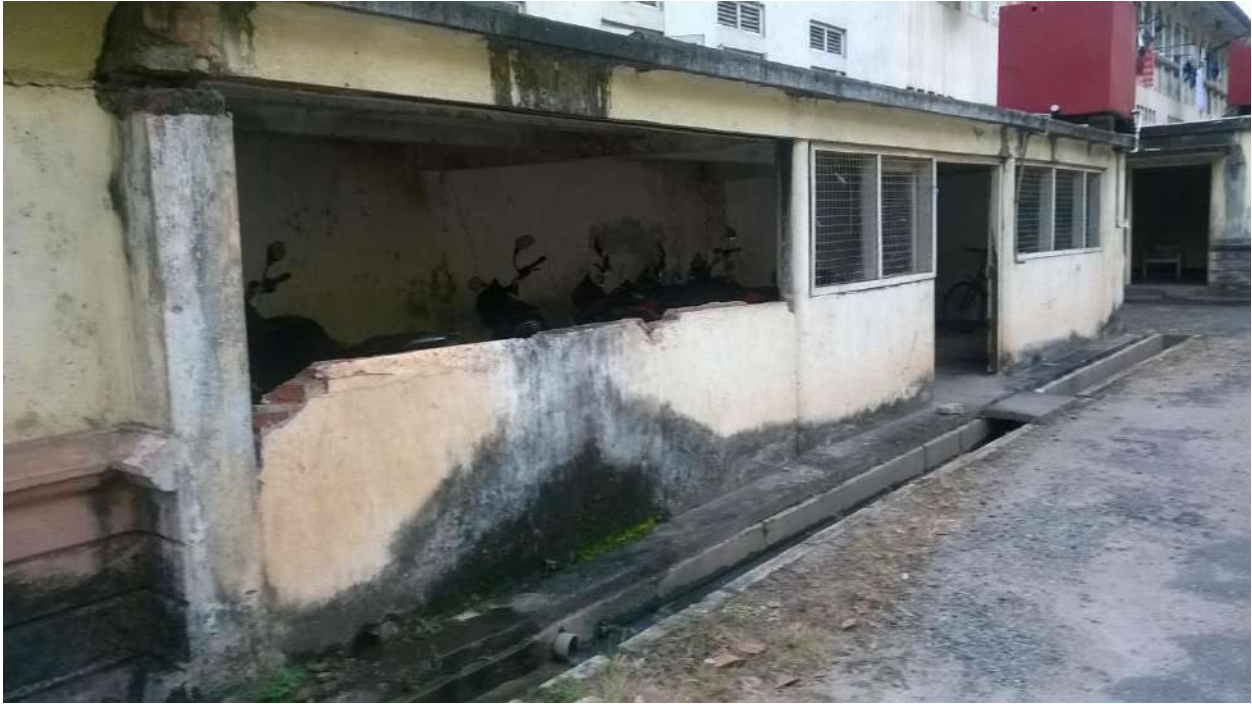
Existing cycle shed
