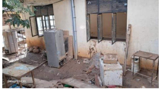
Damaged Refrigerator and Freezer - Canteen
