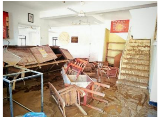
Inside the Canteen after the Flooding
