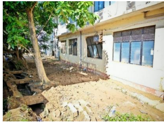
Rear View of DFAPH
