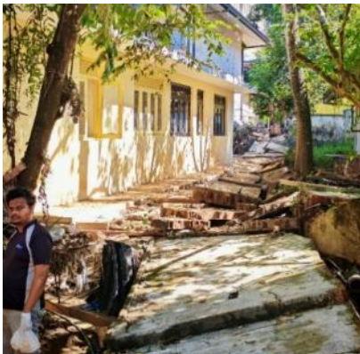
Rear View of DFAPH
