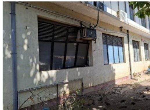
Rear view of DFAPH
